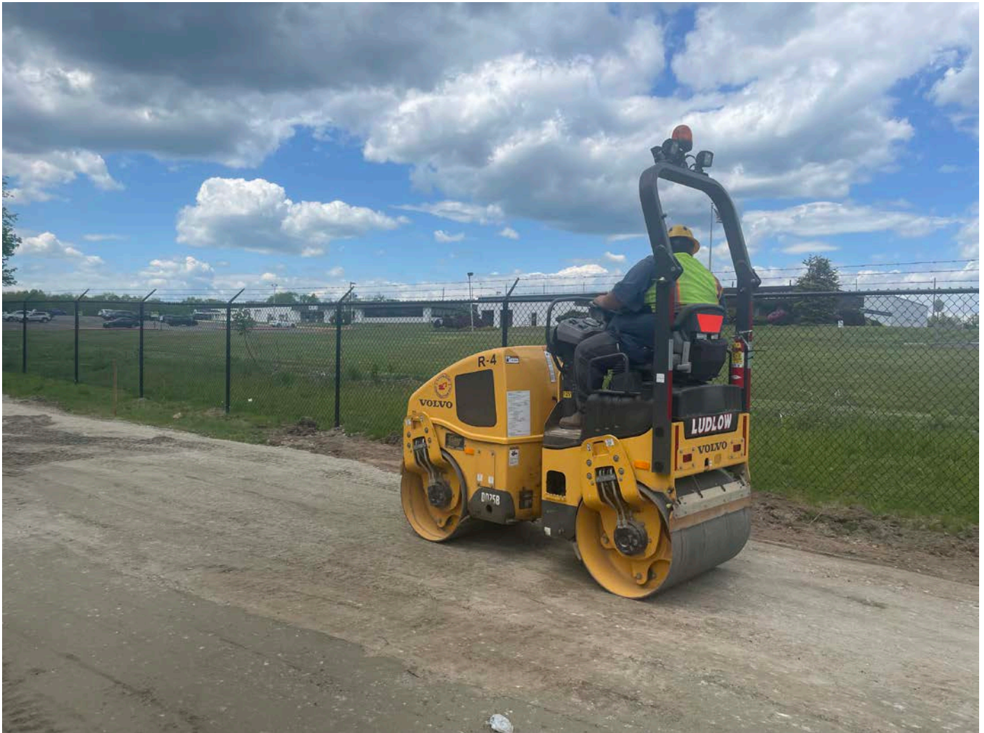
Picture 9: Ludlow compacting the fill on the north side of the Booster Station prior to paving. S. Main Street, Middletown; view to the northwest.
